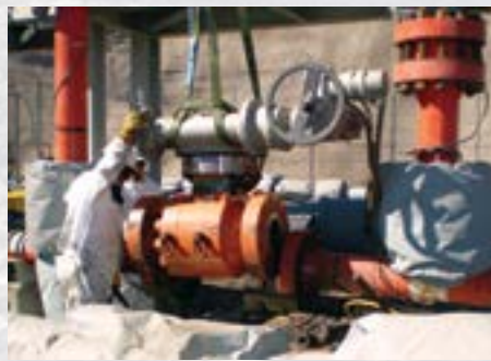
Valve removal for inspection.
