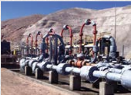
Accuseal 8-inch, 1500 ASME Class critical service ball valve in choke station pipeline for copper concentrate in Chile.
