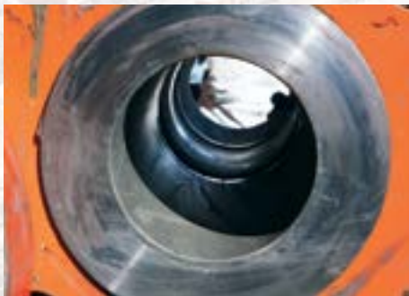
View through downstream bore, open position.
